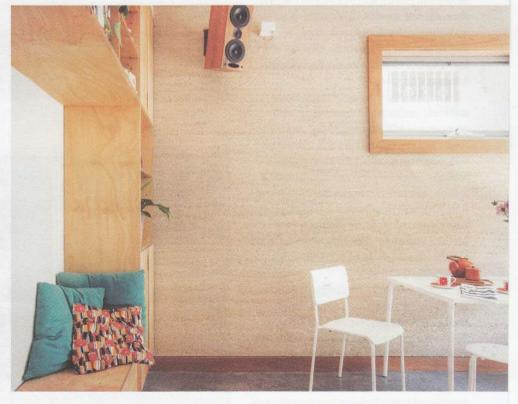
A hempcrete walling system was chosen for its highly insulative properties and consists of hemp, sand, lime and a 'secret' binding agent. An acoustic rating of Rw 47 (the weighted sound reduction level) was required due the house's location on a flight path – the 125mm of hempcrete insulation yields Rw values in the mid 50s.
