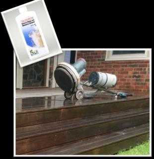
Using the Glouros prior to oiling will remove any fungi/dirt and greying from the weathered timber.
