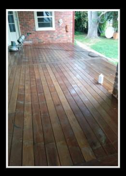
Once wet, use a stiff brush, broom or a buffing machine with a white pad underneath to clean/ scrub the deck.
