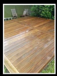
Saturate the surface thoroughly before using the high pressure hose and cleaner.
