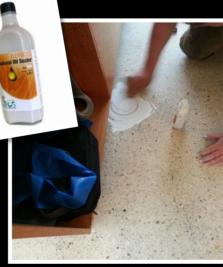
For repairs, work oil in with a fine sand paper over the damaged area
