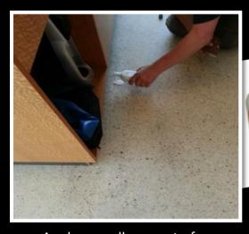
Apply a small amount of the oil originally used directly on the surface, in this case Kunos white
