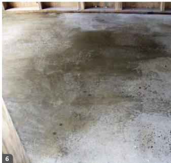
How much grinding needs to take place will be dependent on the requirement of the final look and the condition the concreter has left the slab in.
