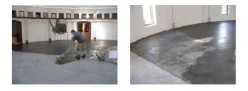
Day 2-Kunos Natural Oil Sealer #244 (Day 3 if humid or cold) Stir well. The second oil coat can be applied, thinly. Repeat steps for 1<sup>st</sup> coat. Leave the oil on the surface for approx 20 minutes to saturate before removing excess as above. <u>If left too</u> <u>long it may start to become tacky</u>. If this happens, work in some more oil to dissolve it again and wipe off. Leave overnight.
