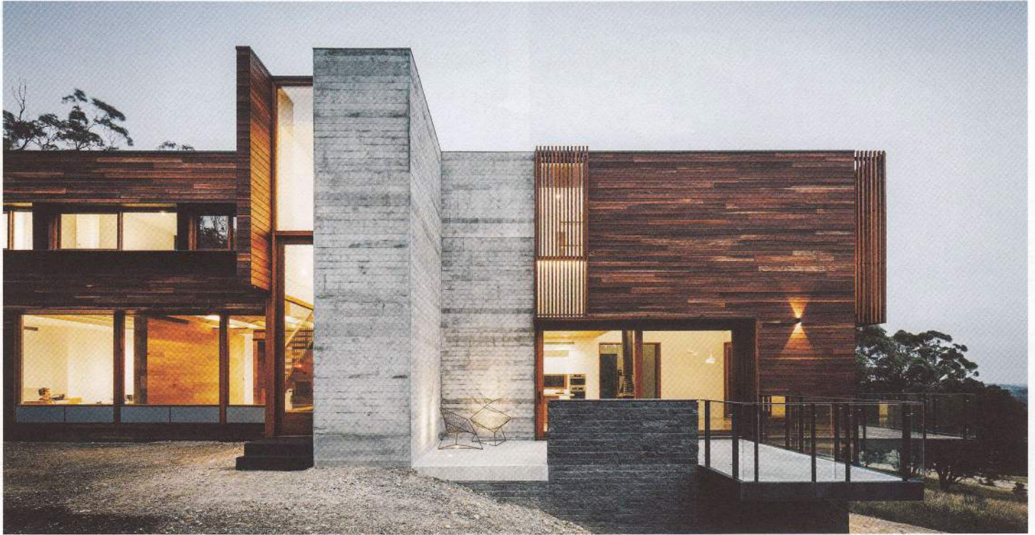
By orienting the house east-west every room gained solar access. opposite page The house cantilevers dramatically over a steep hill to capture views over Ballarat.
