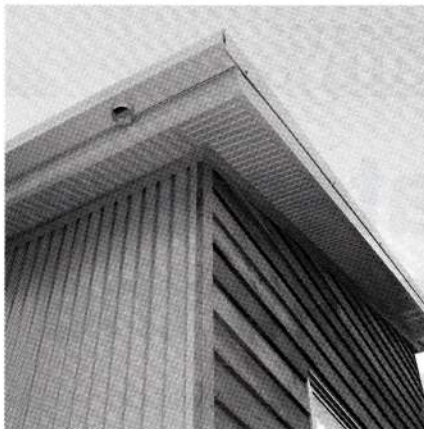
Above left: The absorption pit in all its glory. Above right: Many different materials requires a lot of attention to detail at join areas.
