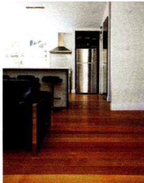
↑ This floor in Auckland, New Zealand, features a coat of Bona Prime Intense and two coats of Bona Mega Extra Matt finish.
