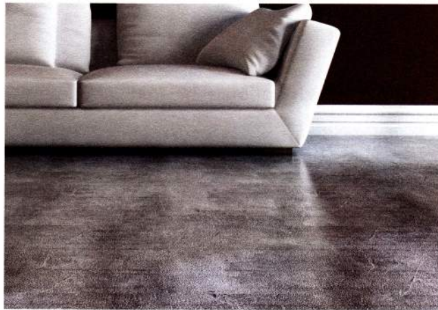
ⓘ An EpiMax professionally finished concrete floor. The finish is achieved with a combination of a solid base colour, a second coat applied intermittently by squeegee and then a clear, non-yellowing seal coat.
