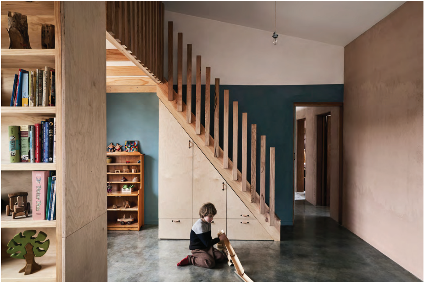
The children's room features twin staircases against each side wall leading to a sleeping loft above the play space; storage is tucked underneath. The concrete slab floor was burnished and oiled with natural oils. Image: Leon Schoots
