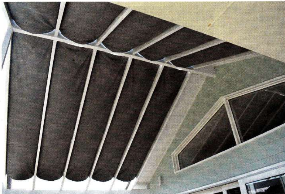
↑ The custom-made canvas cover attaches via stainless steel press studs to the underside of the clear roof of the deck to exclude summer sun; they take it down in winter.
