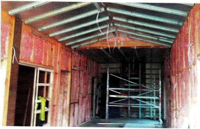
↑ Insulation installation in walls and ceiling.
